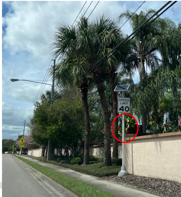
Figure 4 – Missing “YOUR SPEED” Sign - SB Direction
