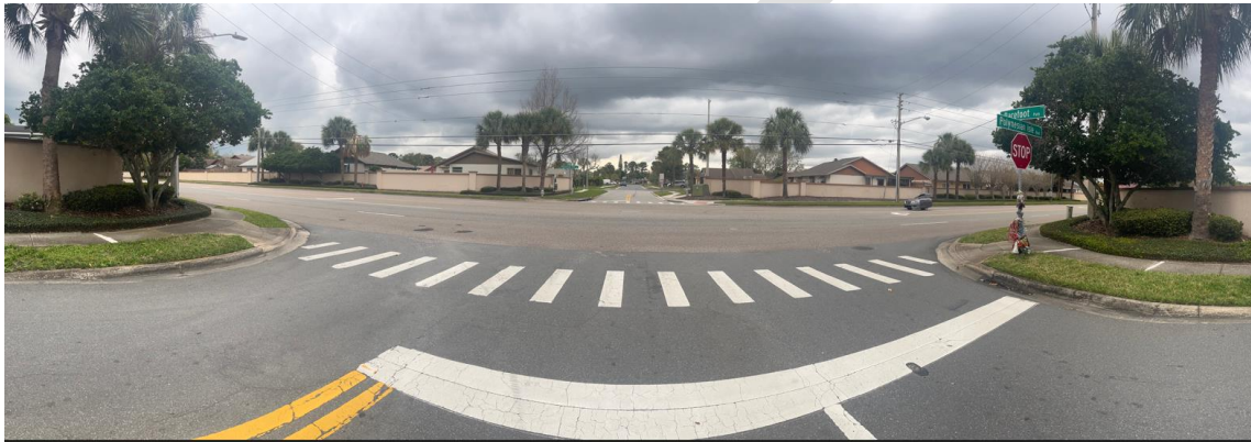
Figure 6 – Reduced Sight Distance WB Approach
