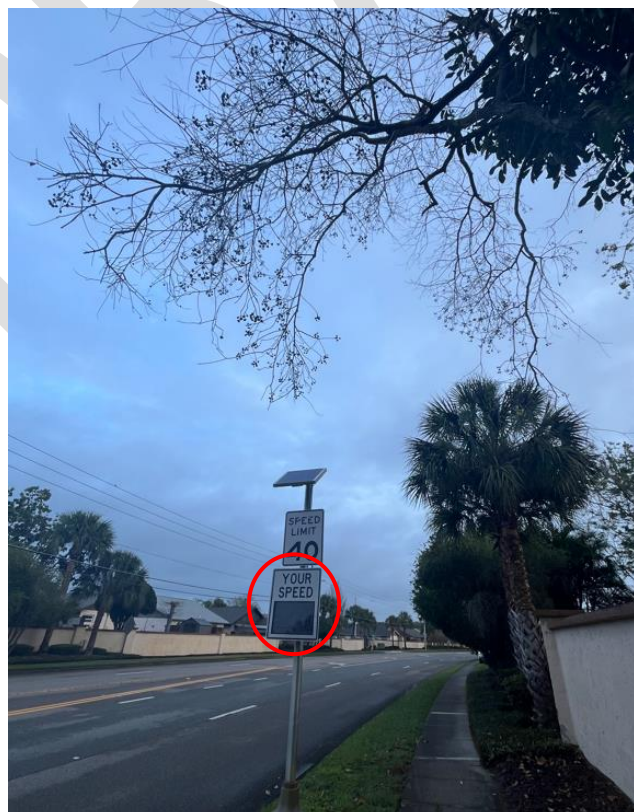
Figure 5 – Inoperational “YOUR SPEED” Sign - NB Direction
